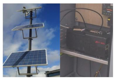
Eddie Broadley of SICE UK described the development of Collaborative Autonomous Power Systems (CAPS) for remote electronic equipment. A hydrogen fuel cell was installed in a trial in 2016. The system is modular so it can accommodate future advances and developments. They are developing the refuelling aspect using electrolysis or reformation to produce hydrogen from other materials.
