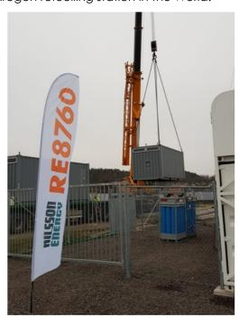
The first container-based RE8760 has been delivered to the hydrogen filling station in Mariestad. This will be powered by the solar park adjacent to it and hydrogen for transportation will be produced electrolysis from water.
